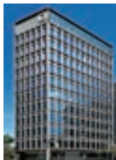
[S-GATE日本橋本町]
